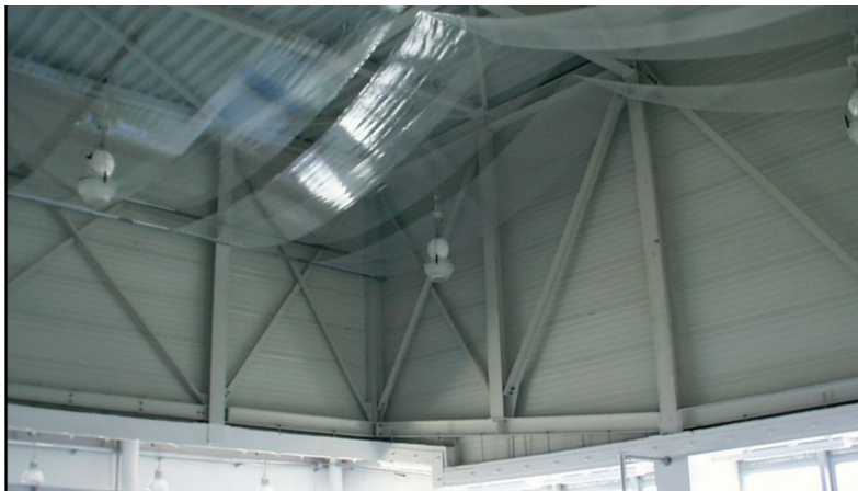
Figure 2.25: Microperforated foil as sound absorber [Wack and Fuchs, 2004].
